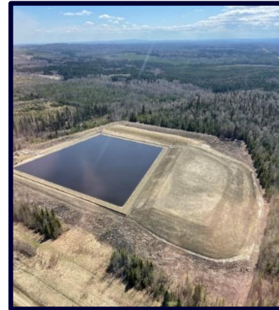
Fresh water reservoir
